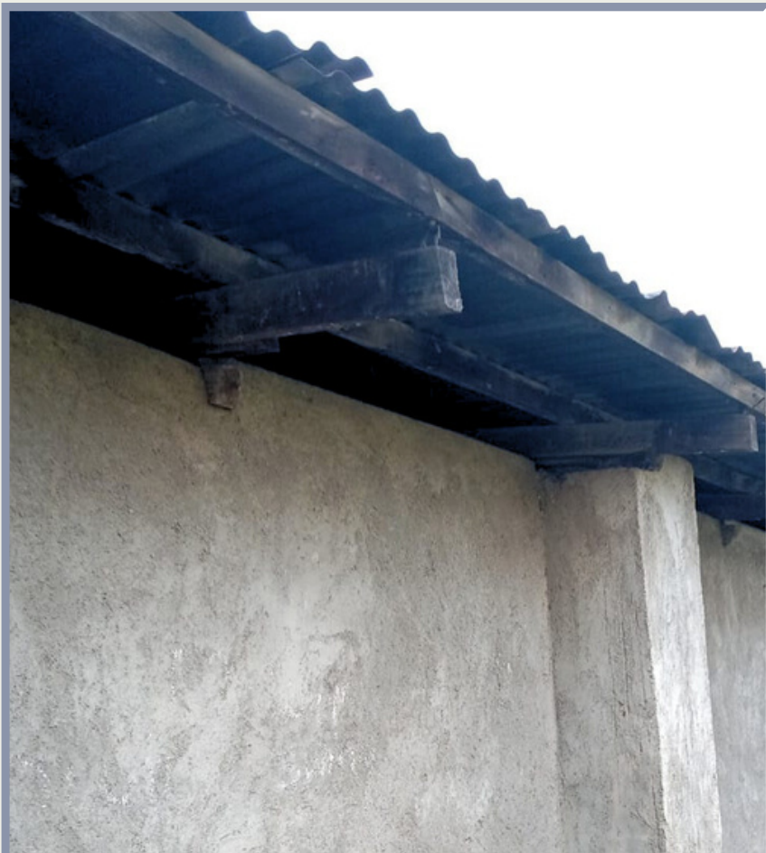
Under the roof and in the rafters
